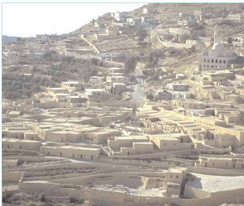
Luxury hotel near Petra Jordan blends into the village and uses vernacular architecture, thick walls, high ceilings, cool water flowing under floors. There are no powered forms of air conditioning or heating - the hotel takes advantage of the natural temperature flux to keep each dwelling comfortable. Note: The lower half of the photo is the 200 room hotel.
